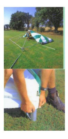
Now place a leg next to each corner and T section. One person then prepares to slot the legs into place whilst the rest of the team lift one side of the marquee.
